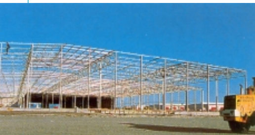
Above: A completed section of the warehouse roof frame
