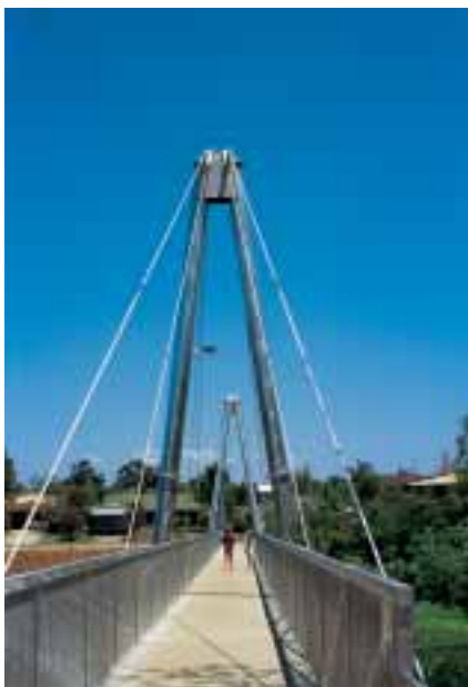
Caboolture River Bikeway Bridge
