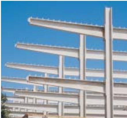
and exits. Decks are split level with long ramps at each end for access from Ground to Level 1, and from then on patrons can use a 'fast up' and 'fast down' ramp system. It is a fully open-deck carpark and fire protection of the steel structure is not required.
