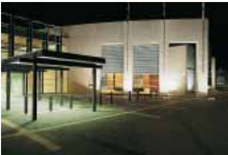
Internal 'street' separating old and new buildings.
