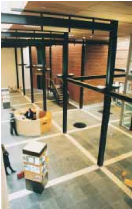
Other areas within the building show off exposed painted steel columns and beams, framing infill panels of glazing or other solid material.
