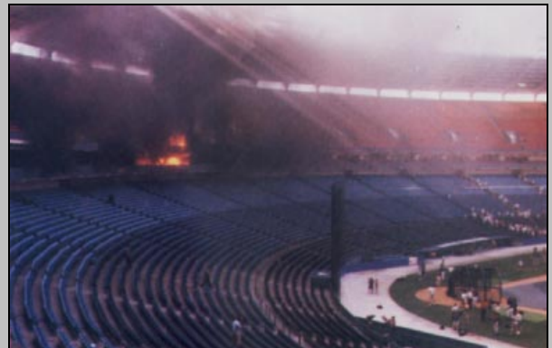
Texas Stadium Fire, USA, 1993 [7]
