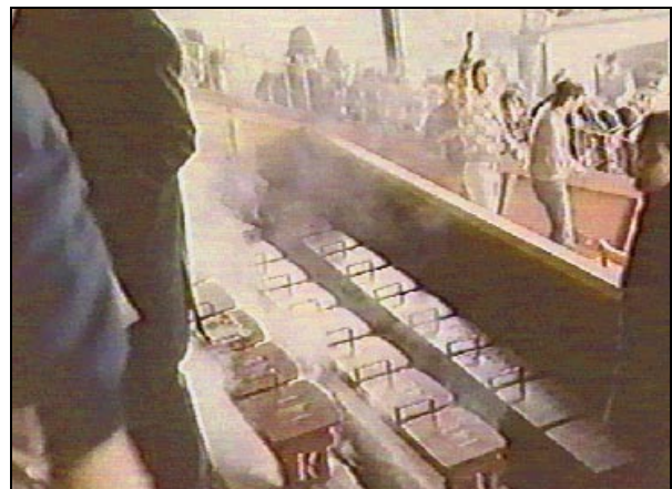
Bradford Stadium: combustibles burning in space below seats
