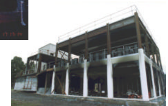
Structure not damaged after test
