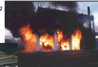
Fire through much of the building
