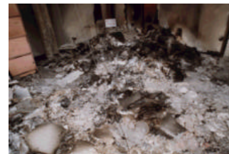
Interior of office after test
