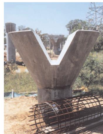
Segments were installed span-by-span (above) or by balanced cantilever. Complex prefabricated reinforcement was required for bridge columns (right).
