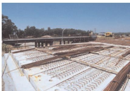
two of his patented mobile steelfixing rigs to place the steel, completing up to 500m of roadway a day.
