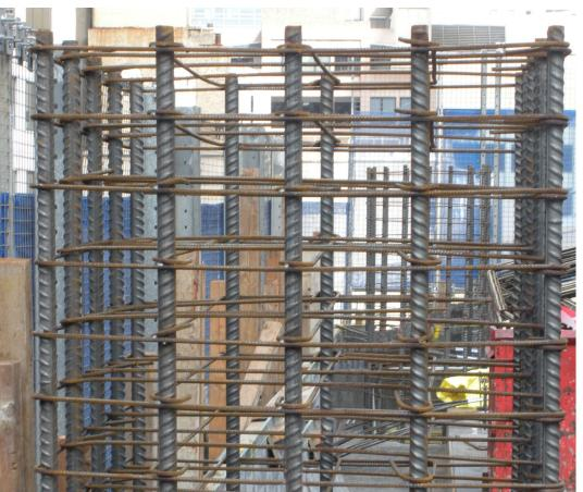
The smaller intermediate beams are fully welded, while the large beams have been specifically designed to have a number of loose bars within the frame. The inclusion of post-tension cables is a unique aspect of the beams. Once the cables are fixed in place, the loose bars are adjusted into the optimum position and manually tied.
