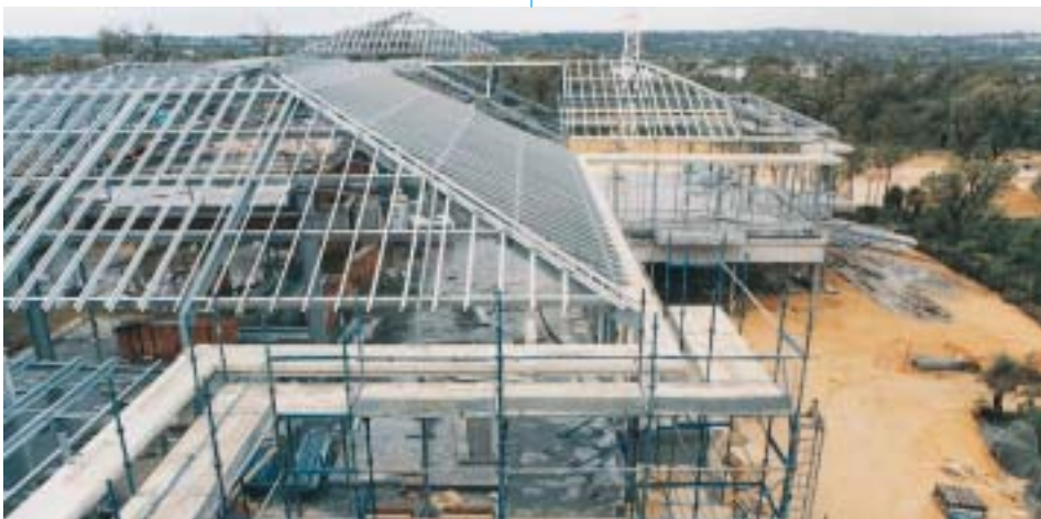
Steel roof framing on Council Chamber.
