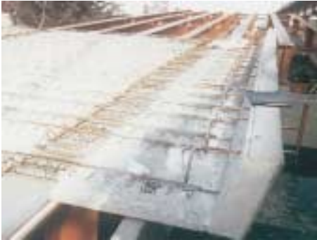
Top: Steel girders in place.
