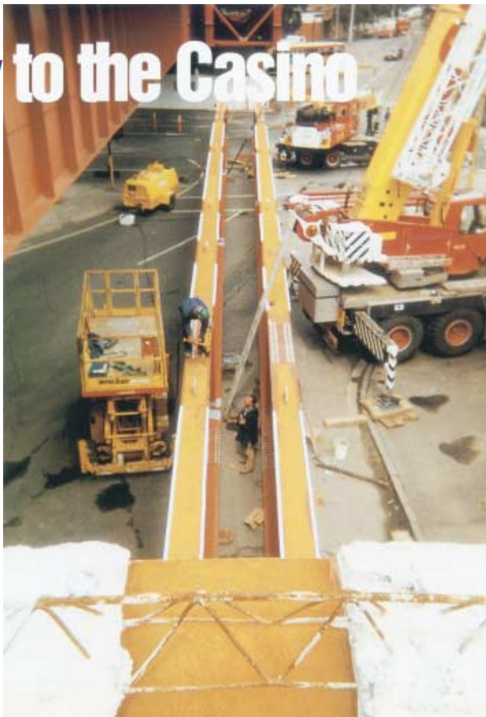
Girder segments being bolted together before lifting directly above.
