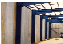
concrete panel wall
