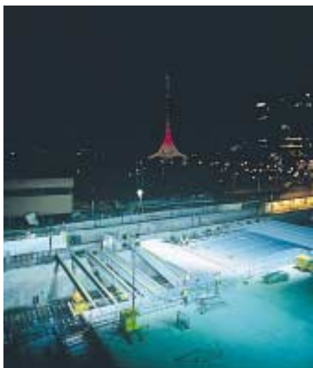
Welded beams being placed during night occupation.
