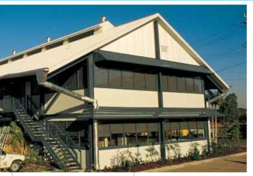
operates in a cross-shop direction at each end of the shop. It also has two 1.5 tonne slewing cranes. The building's roof and walls are clad in Stramit Industries "Monoclad" Colorbond "Off-White". Natural lighting is enhanced by the inclusion of one sheet of translucent fibreglass roof sheeting in each bay. Both the walls and roof have an off-white Colorbond finish to reflect heat and to present a low maintenance finish.
