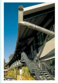
and two storey, 310UB40 exterior columns which are exposed outside the wall line. 150mm thick reinforced concrete slab on "Condeck" profiled steel decking comprises the floor structure which is in turn supported by continuous 360UB45 beams over the internal support. Beams are composite with the slab and are spaced at 4m maximum centres. The floor slab is reinforced with an 1800mm wide strip of F818 fabric top reinforcement over the beams and F62 fabric generally throughout.
