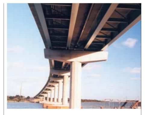
metre footway, plus steel crash barriers and pedestrian railings. Total width is 10.8 metres. The superstructure comprises four steel I-Girders topped by a 200 mm thick reinforced concrete slab and 50 mm of asphalt. Suspended below the deck is a 300 mm diameter water main.
