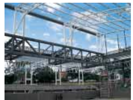
Roof trusses spanning the pools.
