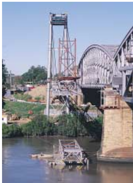
Left: Construction of the new bridge adjacent to the Heritage Listed Albert Bridge.
