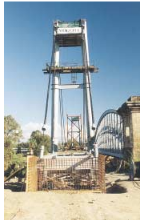
Tower and deck during construction.
