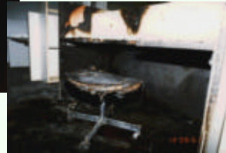
Extent of damage after test
