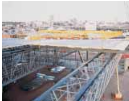
Panelised roof construction.
