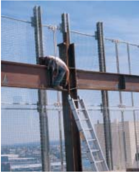
Erection of perimeter beams.
