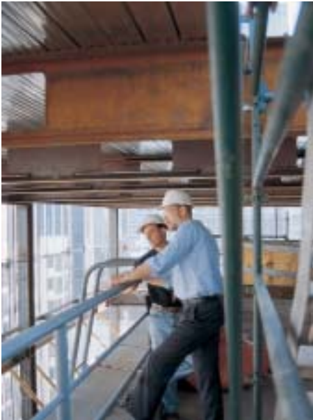
Steelwork on Level 16, showing web penetrations.
