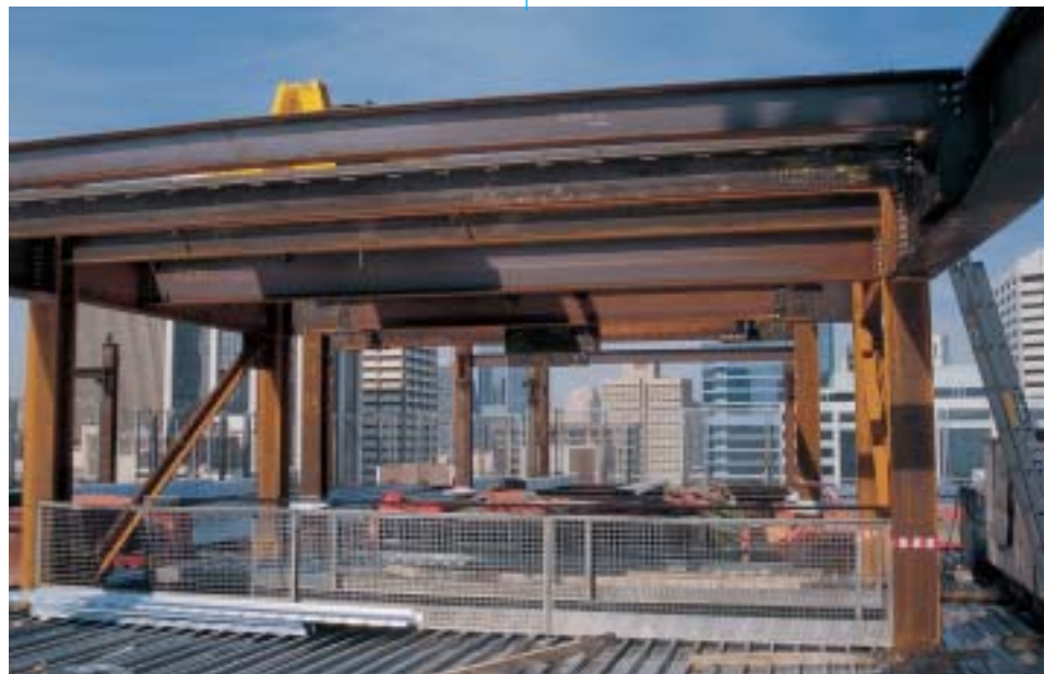
Diagonal bracing indicated core location.
