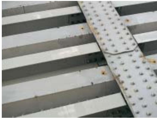
Figure 1. Glenelg Street bridge, showing additional strengthening beams.
