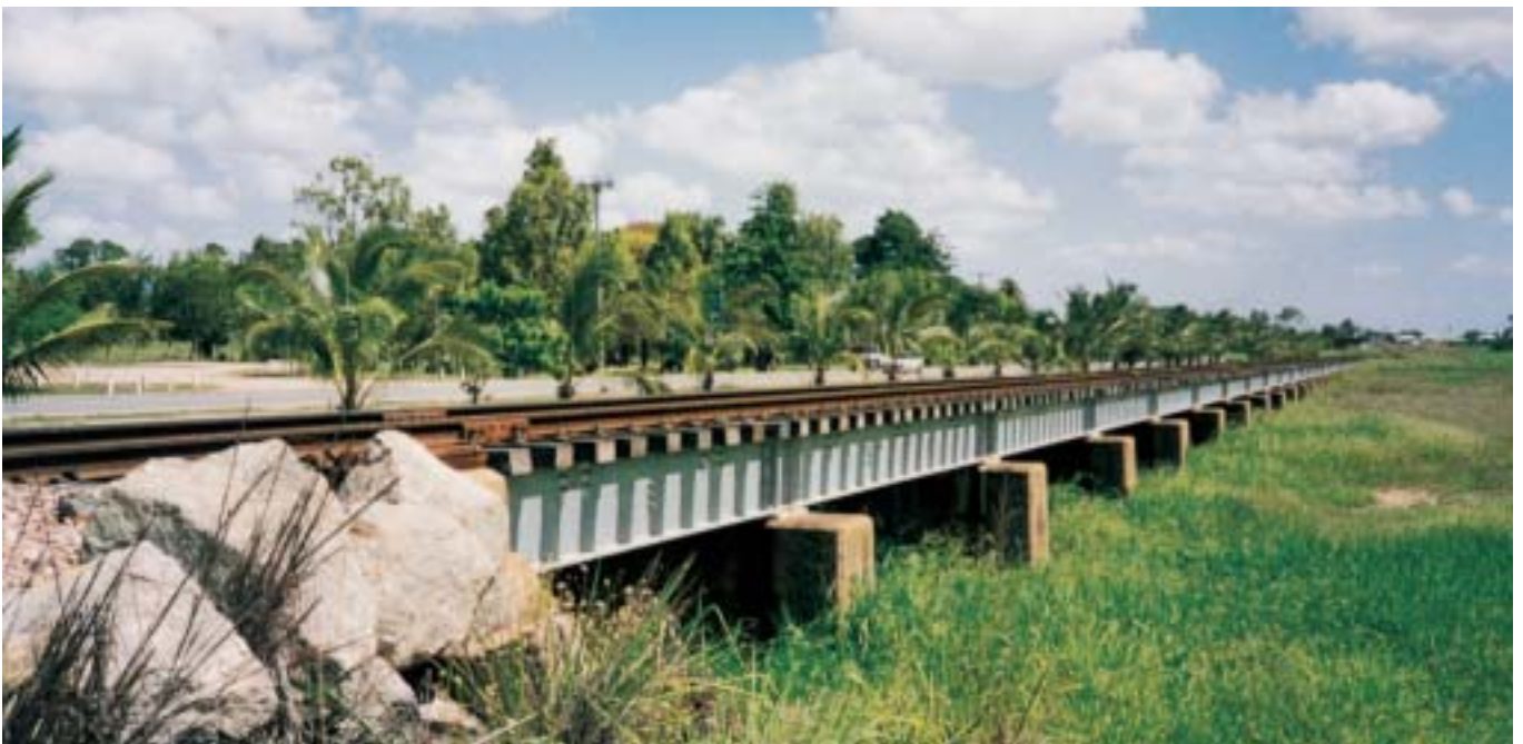
Figure 14. Plantation Creek bridge.
