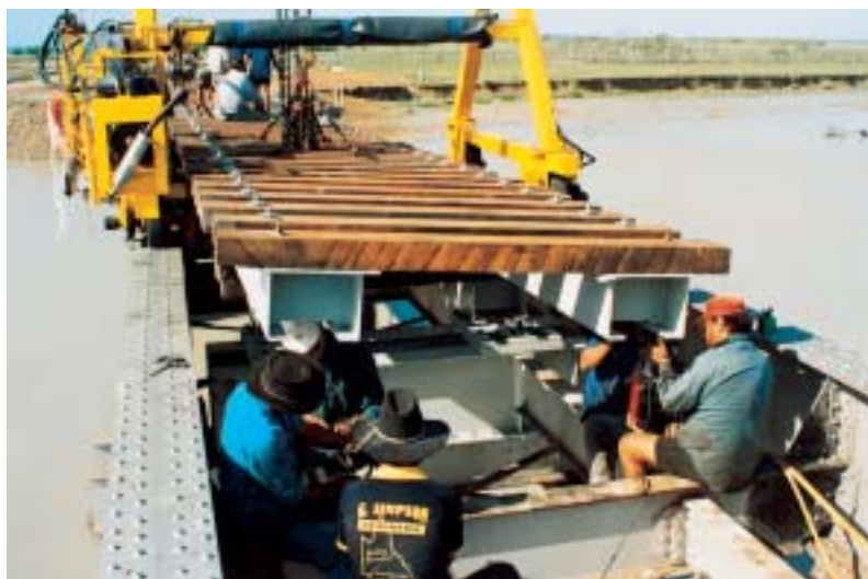
Figures 12 and 13. Erection of new spans from travelling gantry at St Lawrence Creek bridge.
