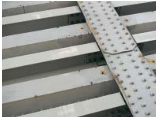
Figure 1. Glenelg Street bridge, showing additional strengthening beams.
