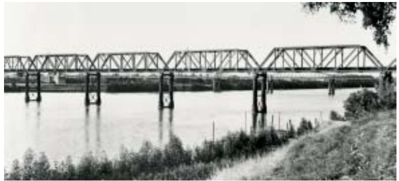
Figure 7. Erection of new girder spans at Murray's Creek bridge.
