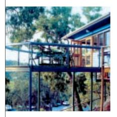
The dimensional accuracy of the steel frame enabled pre-fabricated wall and glazing panels up to 4 metres in width to fit easily and accurately within the steel members, and provided an inherently stiff and structurally efficient main frame structure for the floor, wall and roof structures.
