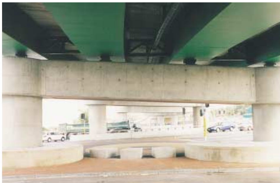
Bridge pier cross head modelled on steam engine crankshaft.
