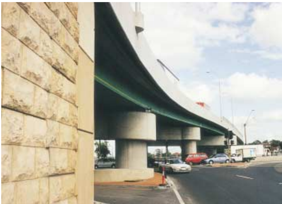
Curved girders with paintwork reflecting rail heritage.
