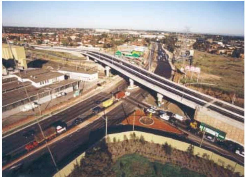
The new Roberts Road bridge.
