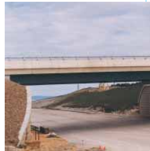
Majors Road bridge
