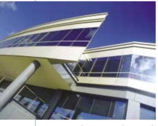
compartment with extensive use of unprotected steel beams in both the office space and the carpark. An estimate of the savings on the erected steel cost was in the order of 8%, as a result of using unprotected steel beams.
