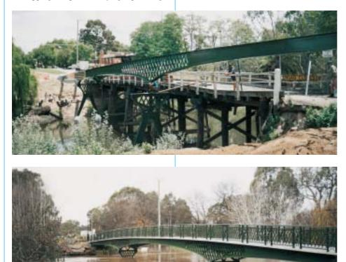
practical advantage of simplifying the boilermaker's task of cutting and fitting. In the lattice regions flat bars 30 degrees to the vertical were fitted and butt welded between the stems of the T's. Steel angles, 30 degrees to the vertical in the other direction, were placed on the inside faces, overlapping the stems of the T's and fillet welded. Care was taken in the welding specification and sequence to minimise distortion.
