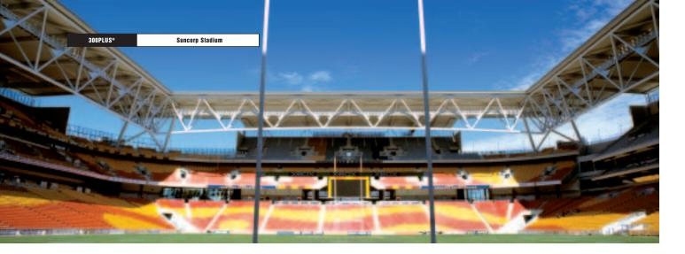
The design of the roof and grandstand structures used innovative engineering features to reduce the weight and cost of the structural steelwork, and facilitated rapid and safe erection of the roof.
