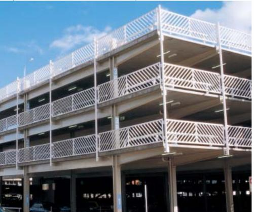
the columns at the grid spacing noted above and in accordance with the requirements of A82890.1 SAA Parking Code. Bracing members were aligned with the ends of parking bays.
