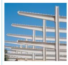
and exits. Decks are split level with long ramps at each end for access from Ground to Level 1, and from then on patrons can use a 'fast up' and 'fast down' ramp system. It is a fully open-deck carpark and fire protection of the steel structure is not required.
