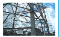
In order to give the sheets of HANDIMESH additional support, 7 x 2mm high tensile wires (4 outside and 3 inside the tower) were attached and tensioned to the underside of the mesh.
