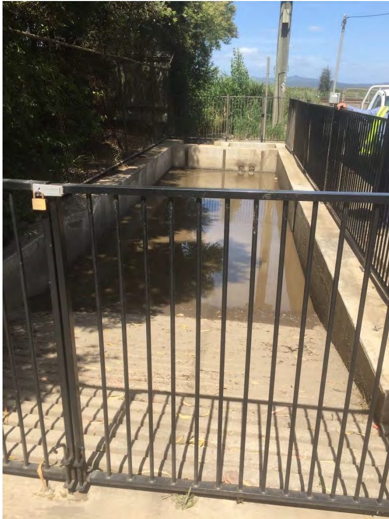
Photo 7 – Stormwater collection system – Gross pollutant trap.
