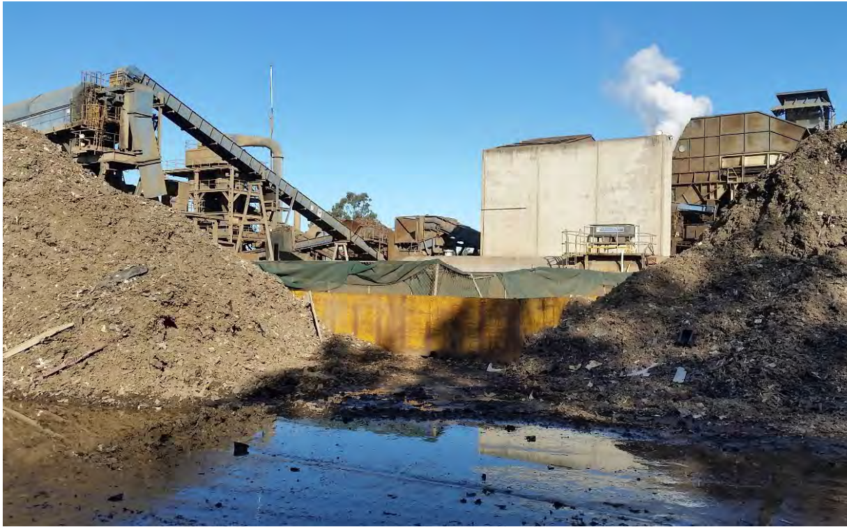
Plate 1 Shredder Yard First Flush Pit
