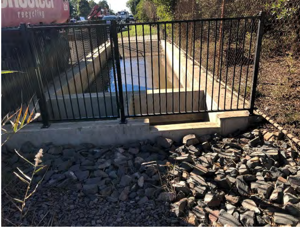
Plate 1 Internal Roadway Sediment Trap
