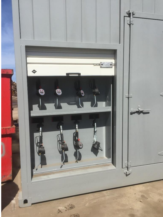
Photo 1 – New bunded facility for storage and dispensing of oils.
