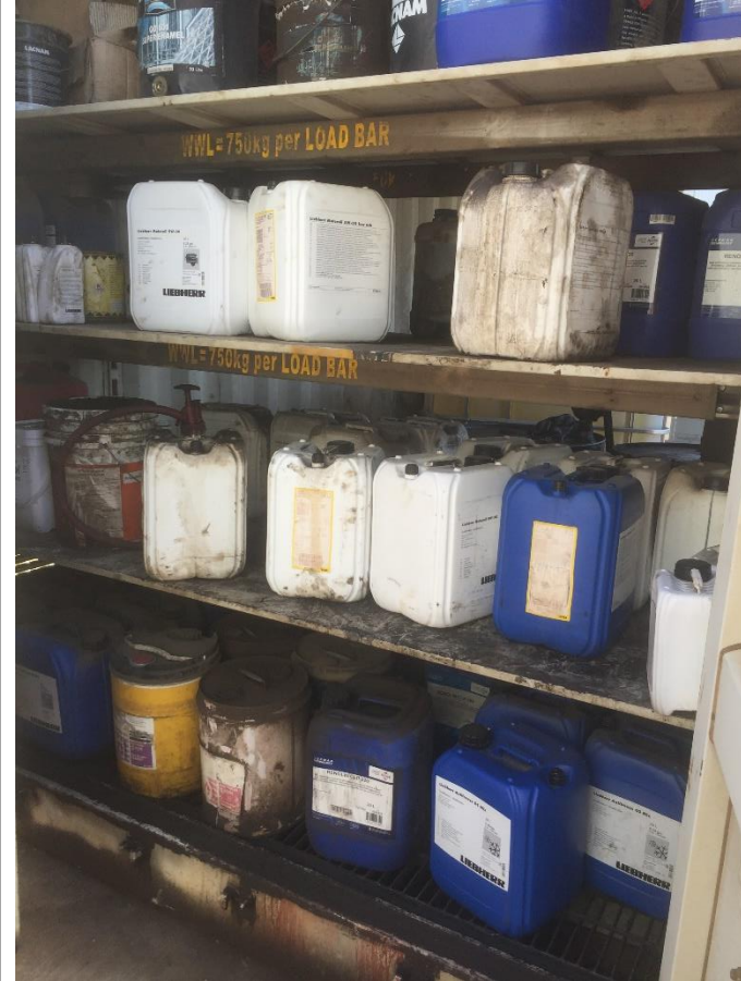
Photo 2 – Oil containers in bunded container.
