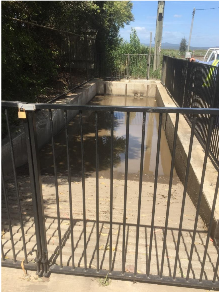
Photo 7 – Stormwater collection system – Gross pollutant trap.
