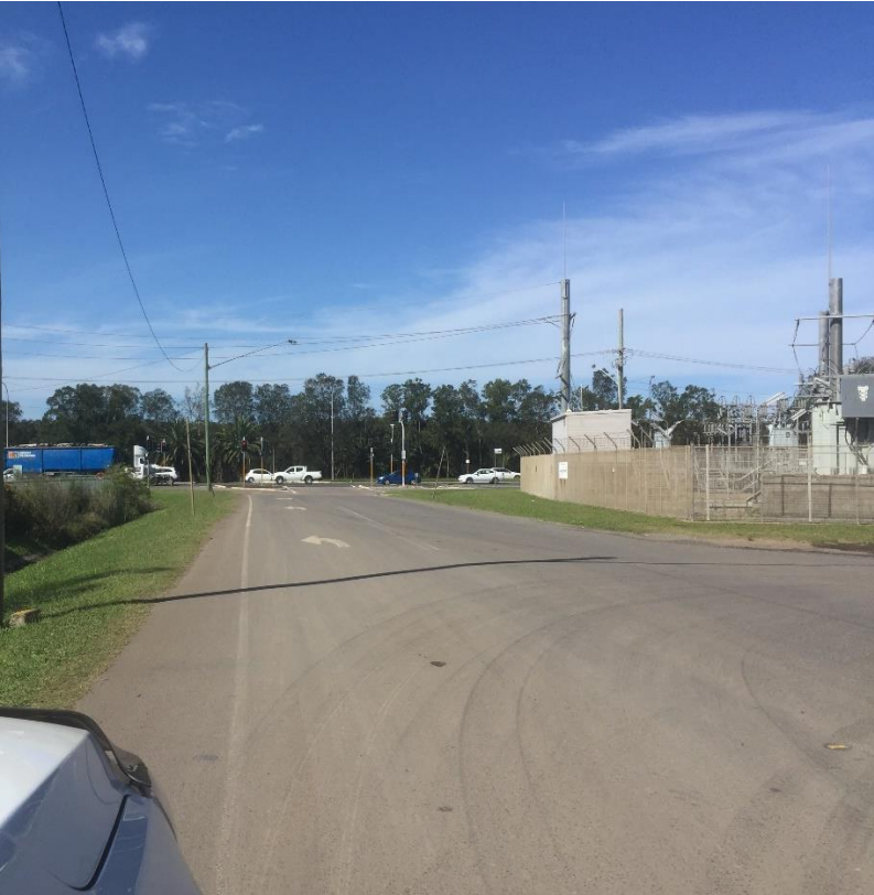
Entry/ exit to Pacific Highway
