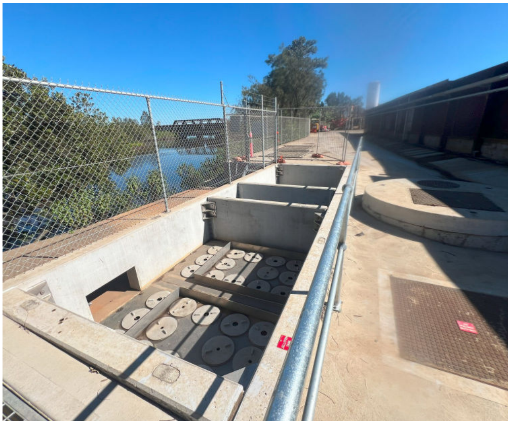
Plate P2. Internal stormwater management system
