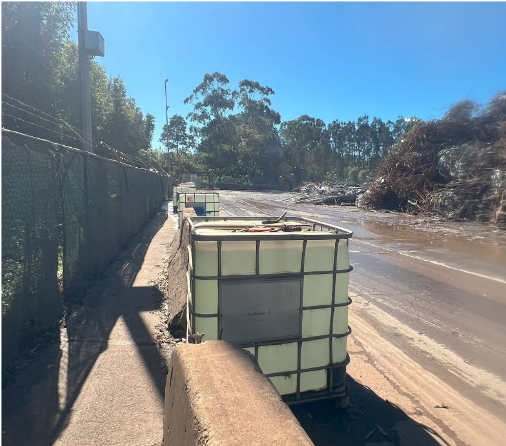
Plate P9. Water storage for fire management in the shredder yard
