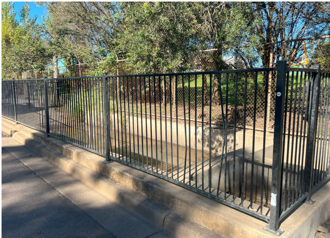
Plate P6. Stormwater management system (Sparkes Street)
